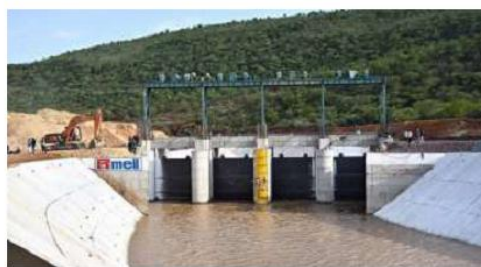
Once fully operational, the project will provide drinking water for 23 lakh people and irrigation for 4.47 lakh acres. SPECIAL ARRANGEMENT
